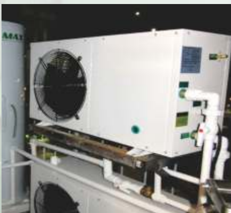
DOMESTIC 60°C HEAT PUMP WATER HEATER
